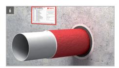
Finally apply the identification sign to the penetration seal. The identification sign must be place next to the penetration seal to the building component and is available at FLAMRO Brandschutz-Systeme GmbH.
