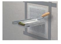
Coat the seal surface with FLAMRO<sup>®</sup> BMA (DFT ≥ approx. 2 mm).
