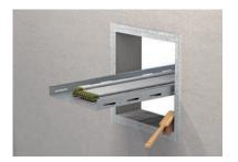
2. Coat the cable and opening with FLAMRO® BMA.
