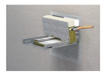
4. Pack the remaining openings with mineral wool or fill with FLAMRO® BMA.
