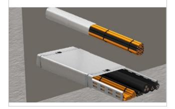
5. If required or mandatory, fill the identification label and apply on the side or below (not on!) the installation. Remove mortar residues from cables, walls and floors. Dispose of cover foils and mortar residues properly.
