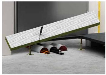
4. Brush the edges of the mineral fibre board using PYRO-SAFE FLAMMOTECT-A and firmly seat board into position. Place the mineral fibre board so that the painted side is showing on the outside.
