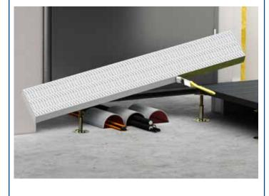
5. Stuff residual opening and expansion joint using mineral fibre. Cut stoppers to size and fit stopper on one side
