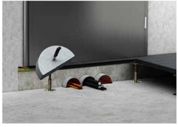
7. Fit stopper on one side and use PYRO-SAFE FLAMMOTECT-A to seal it. Stuff conduit openings with mineral wool and seal with PYRO-SAFE FLAMMOTECT-A.
