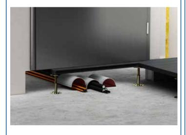
Cut mineral fibre board to size. On the top of the raised floor, approx. 2cm can remain as an expansion joint.
