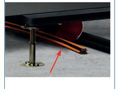
1b. Carefully place the PYRO-SAFE CT ML over the lines.
