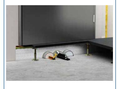
7. Top coat using PYRO-SAFE FLAMMOTECT-A.
